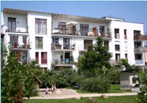
Block associations look after public space in Freiburg
