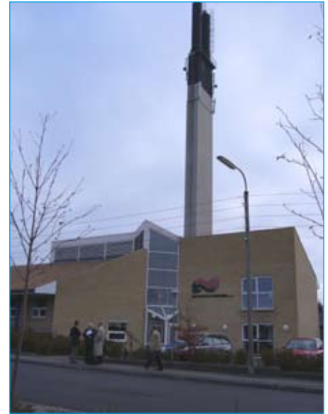
Hoje Taarstrup heating plant and head office. Danish coops help build really sustainable communities
